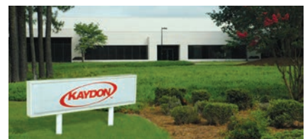
Sumter, South Carolina - Plant 12 B
